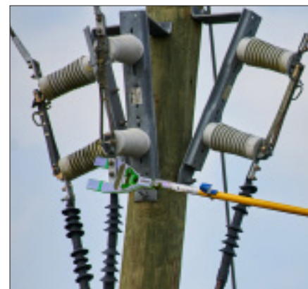
Standard Current Stick on Overhead Switch
