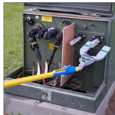
Wide Jaw Current Stick on Pad-mounted Transformer
